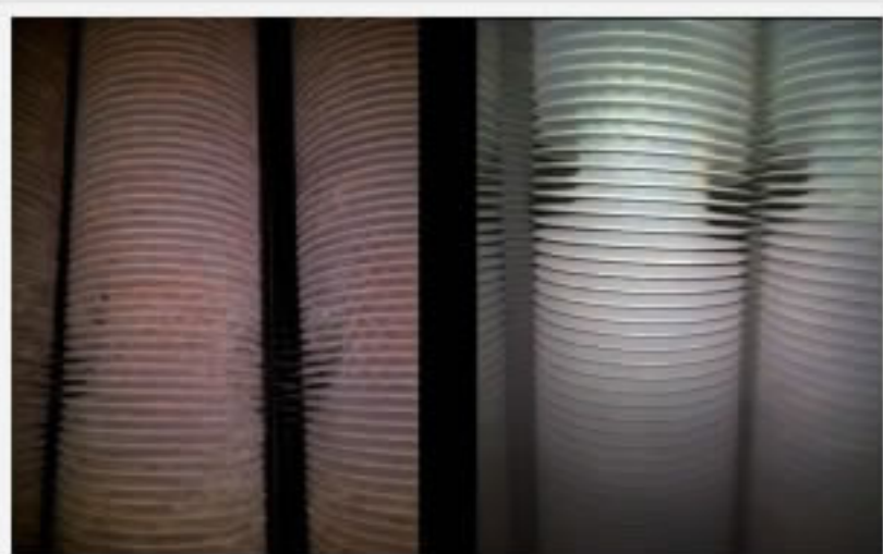
Before and after tube cleaning
