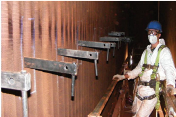
7. Alignment bars are inserted by protected technician to spread tubes and allow deeper penetration of the cleaning wands
