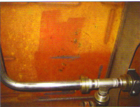
Top: Before the CO 2 cleaning Bottom: After the cleaning, even the burned shop primer has been fully removed.
