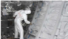
Once traditional insulation gets wet, the material becomes a heat conduit, an odor wick and exposes the metal surface to mild and corrosion. Insulating coatings have no have ability to absorb humidity and cause negative effects, according to Mascoat.
